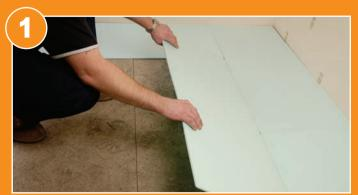
Lay the ECOMAX-LITE Thermal Insulation (available separately) in a "brick work" pattern and fix with adhesive tape.
