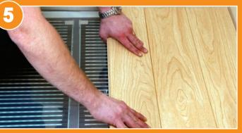
Lay the floor covering as soon as possible to prevent damage to the element.
